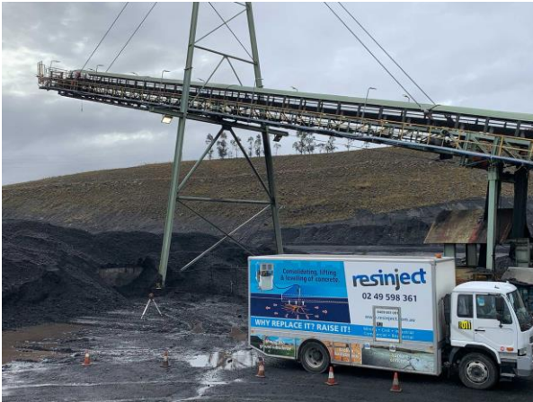
Figure 3. Main Conveyor Trestle Footings
