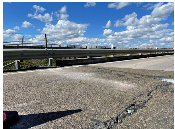
Figure 4. Post-treatment Roadway Surface
