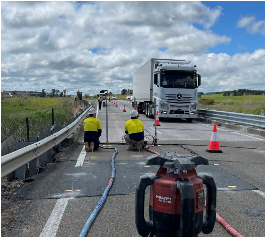
Figure 3. Injection Works Under Traffic Control
