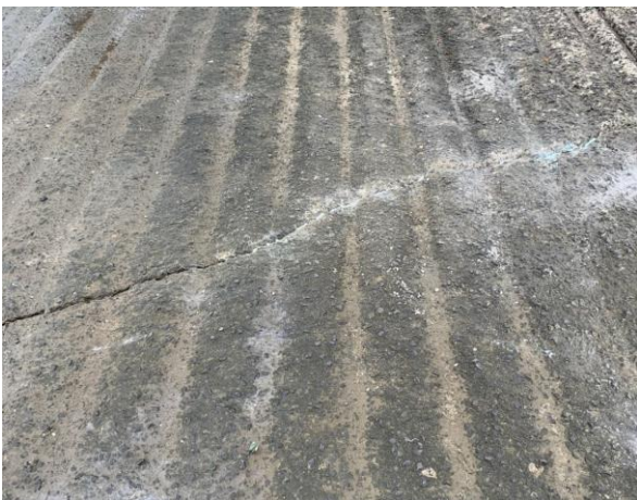
Figure 3: A treated slab which was raised and re-levelled 100mm
