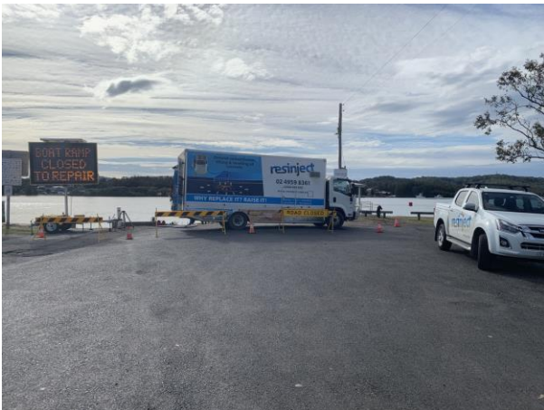
Figure 1: The Resinject Crew setting up prior to works commencing
