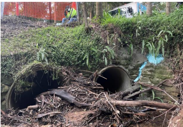
Figure 1: The two culverts underneath the road.
