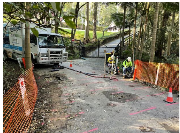
Figure 2: The Resinject Emergency Maintenance crew completing the works
