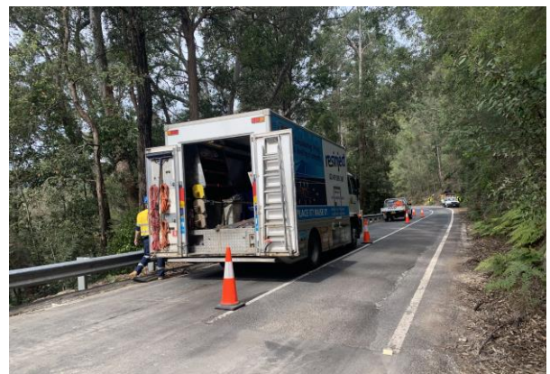
Figure 2. Resinject Crew preparing for the injection methodology.
