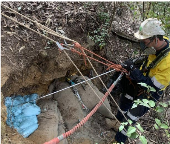
Figure 3. Resinject Team Member Safely Sealing the Adit
