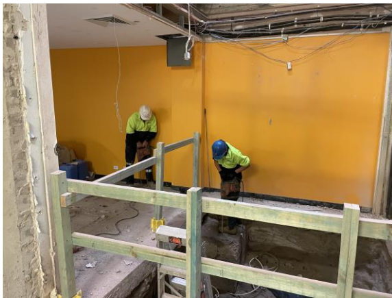
Figure 3: The Resinject Team drilling holes to inject RSJ170 structural resin
