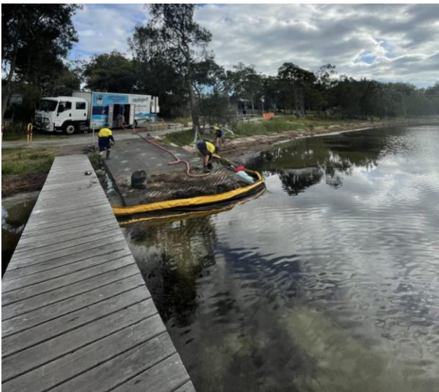
Figure 3. Setting up a damming net to protecting the environment
