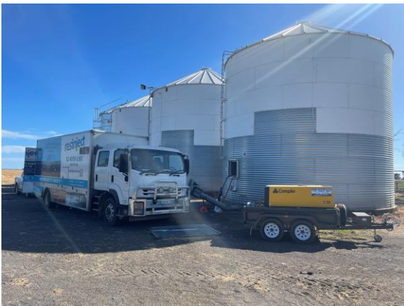
Figure 1. The Resinject Rig outside the three large grain silos
