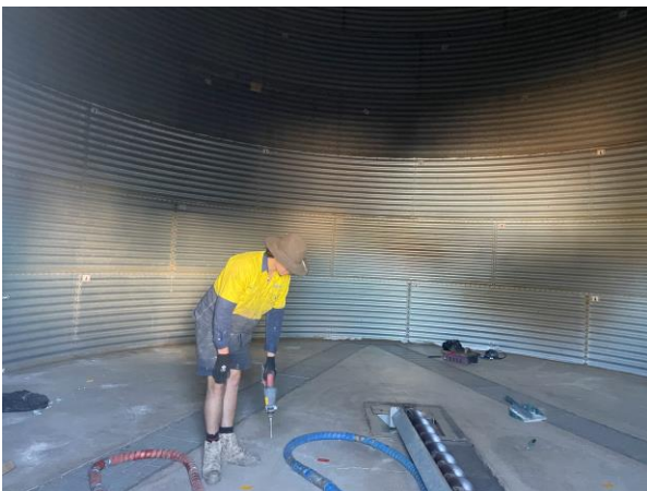
Figure 3. Resin injection process inside a grain silo
