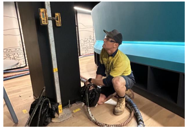
Figure 2. A Resinject operator completing the resin injection methodology.
