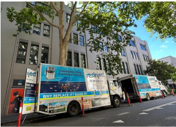
Figure 1. The Resinject Rigs outside the commercial 4-story building
