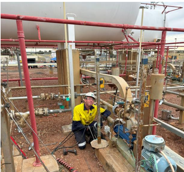
Figure 2. A Resinject operator completing the resin injection methodology
