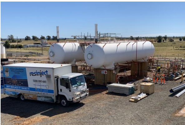
Figure 1. The Wallumbilla LPG Facility
